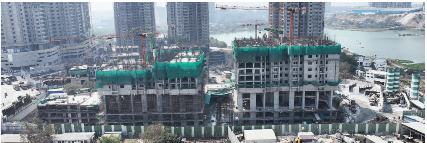
Tower A & B Progress (January, 2026)
