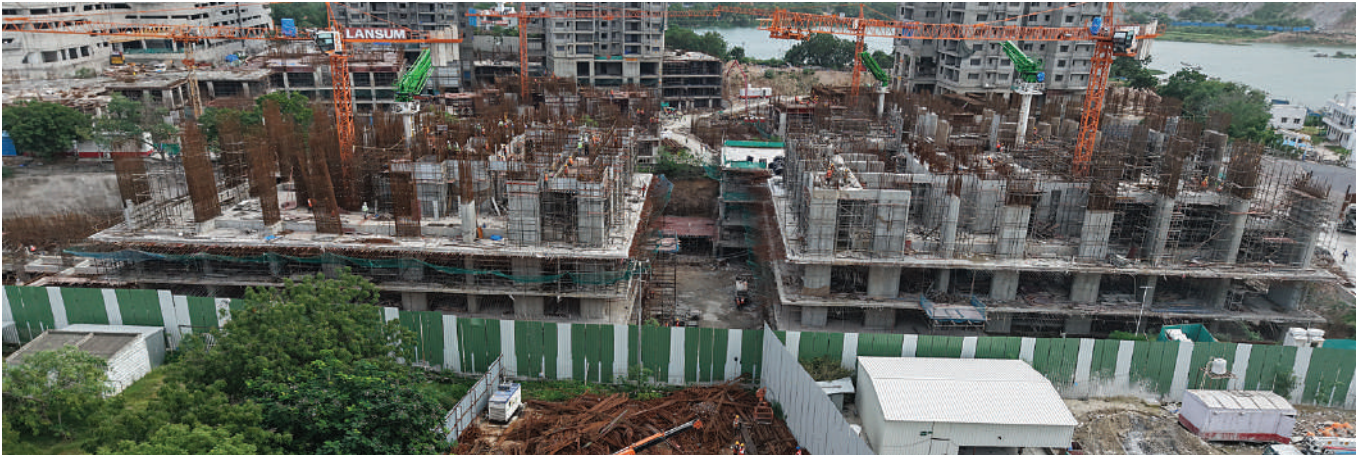
Tower A & B Progress (July, 2025)
