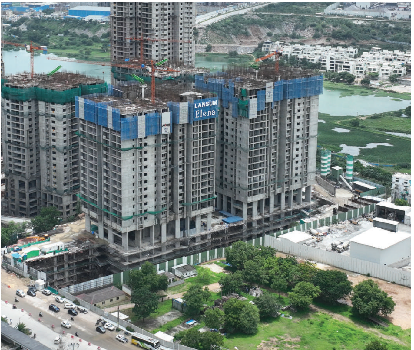
Current Construction Image
