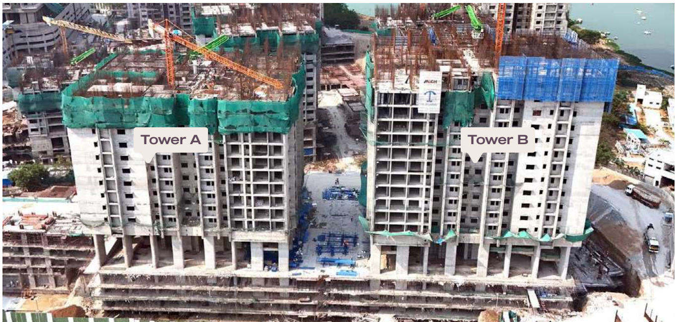
Tower A & B Progress (April, 2026)
