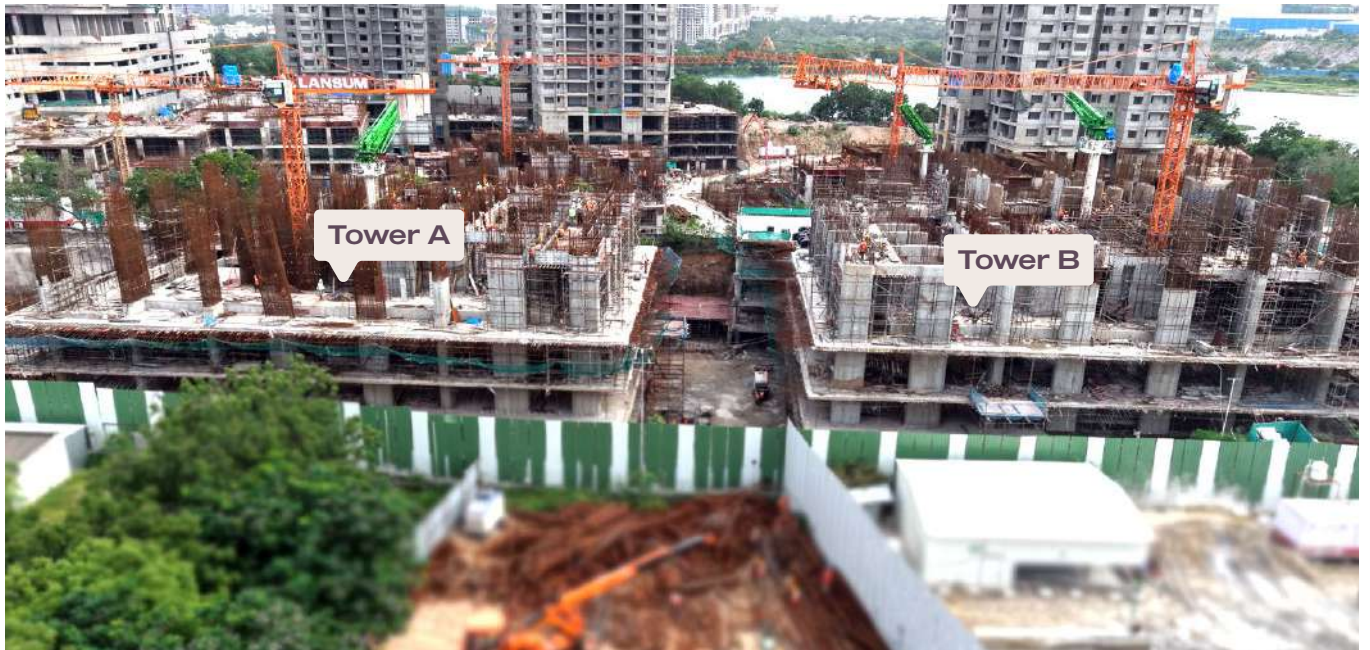
Tower A & B Progress (July, 2025)
