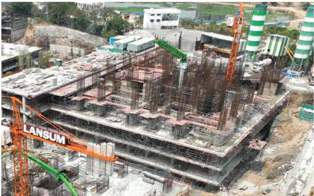
Tower B Progress
